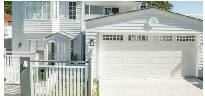
Grange with Stockton windows
